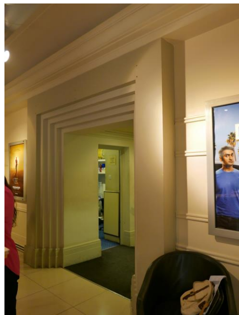
The Entrance Hall at ground floor level and the opening leading down to the two preview-cinemas, showing surviving, original decorative, ceiling and wall plasterwork and veneered doors
