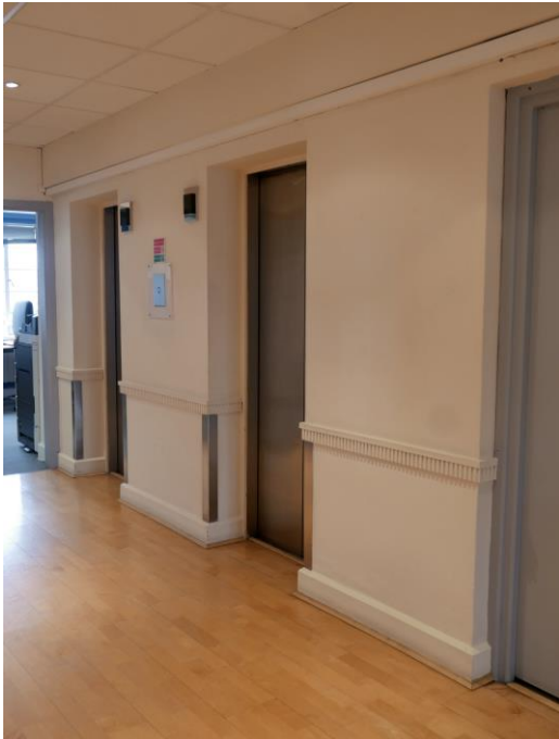
Typical, modernised lift-lobby (at sixth floor level), showing surviving, original, dado-rails and skirtings of Modernistic character, and the original service-lift
