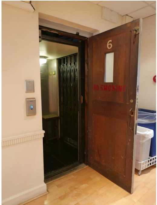
Typical, modernised lift-lobby (at sixth floor level), showing surviving, original, dado-rails and skirtings of Modernistic character, and the original service-lift
