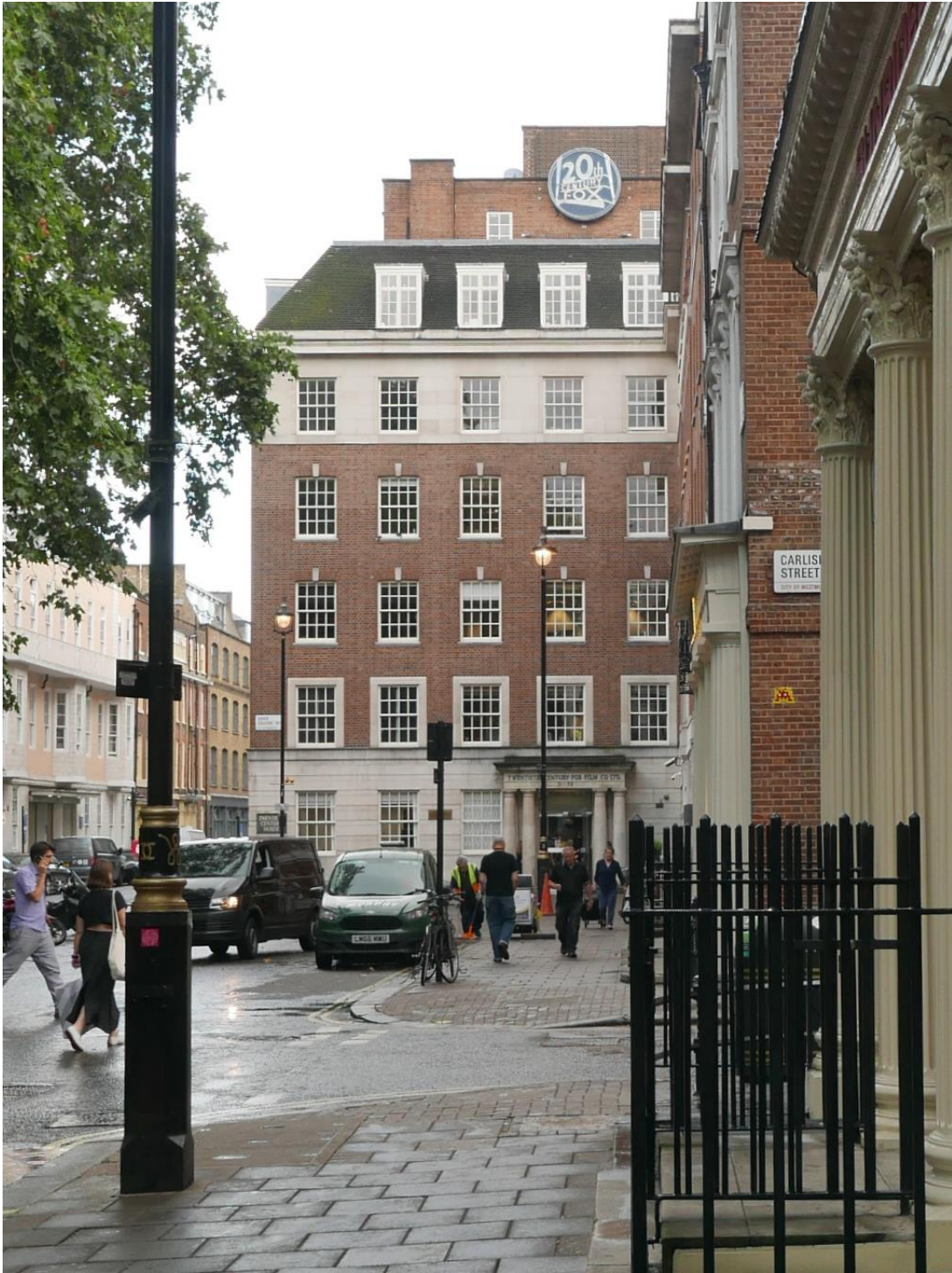
View of Twentieth Century House from the south-western side of Soho Square, showing the surviving, original circular, 20 th Century Fox logo neon-sign at roof-level facing into the Square
