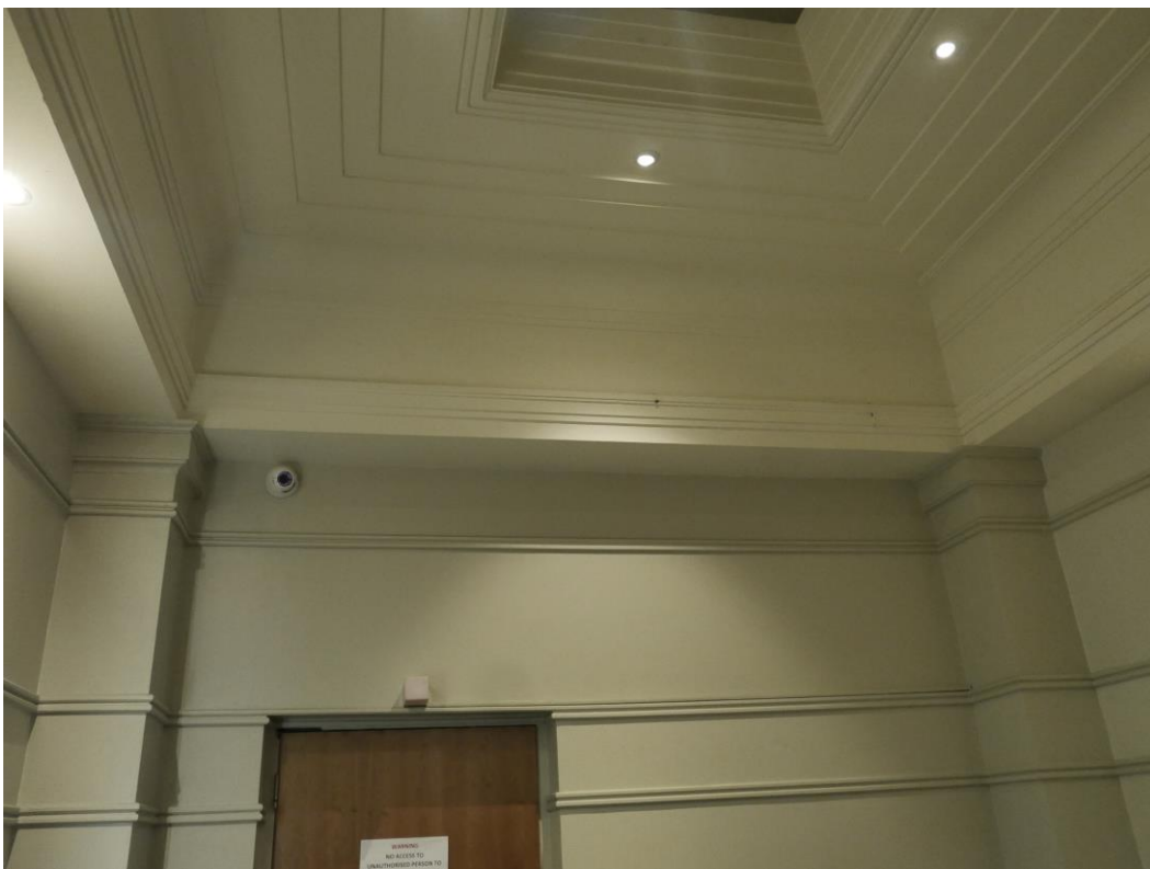
The lobby serving the two preview-cinemas showing surviving, original, decorative ceiling and wall plasterwork
