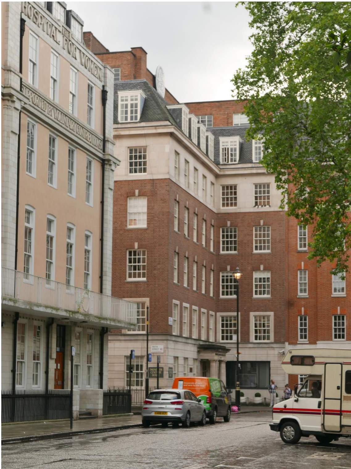
View of Twentieth Century House from the south-eastern side of Soho Square
