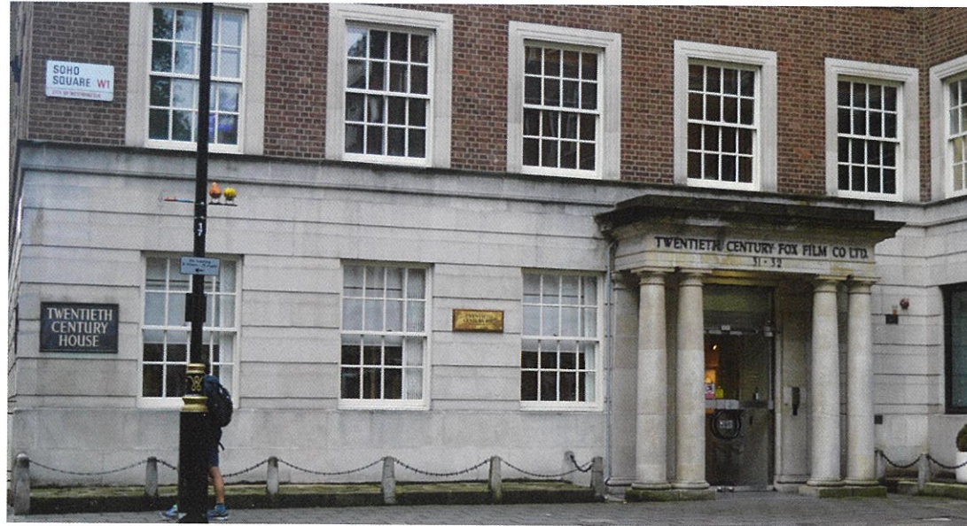
Fig 1 | Existing Portico / Main entrance to the building
