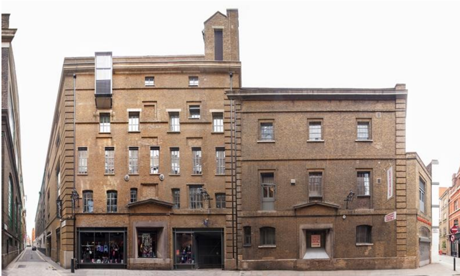
The building on the left and down the street.
