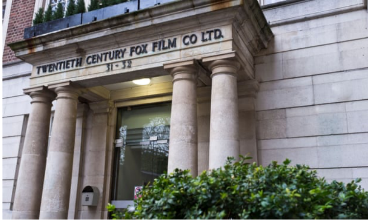
How the building used to look. Photograph: Julie Edwards/Alamy
