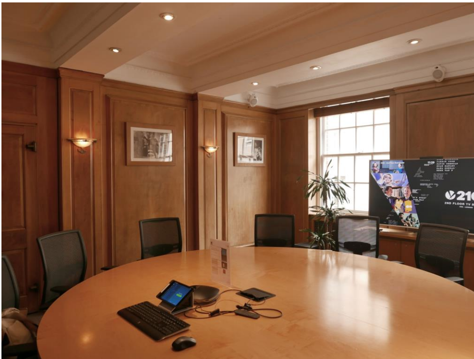
The Board Room at second floor level, showing the surviving, original, full-height, oak panelling and classically-detailed ceiling-cornices
