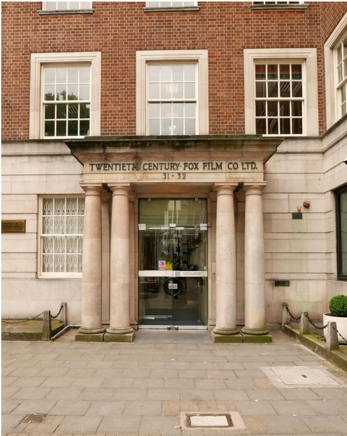
The main entrance to Twentieth Century House: View from the north-west
