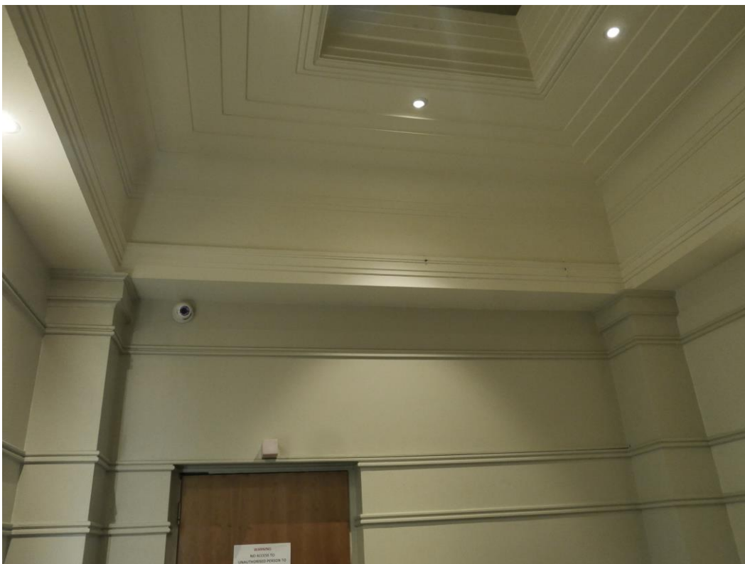
The lobby serving the two preview-cinemas showing surviving, original, decorative ceiling and wall plasterwork
